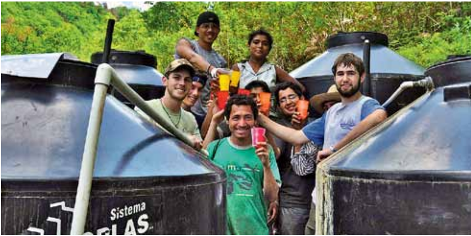
Students work with Honduran villagers to build a sustainable water system.
